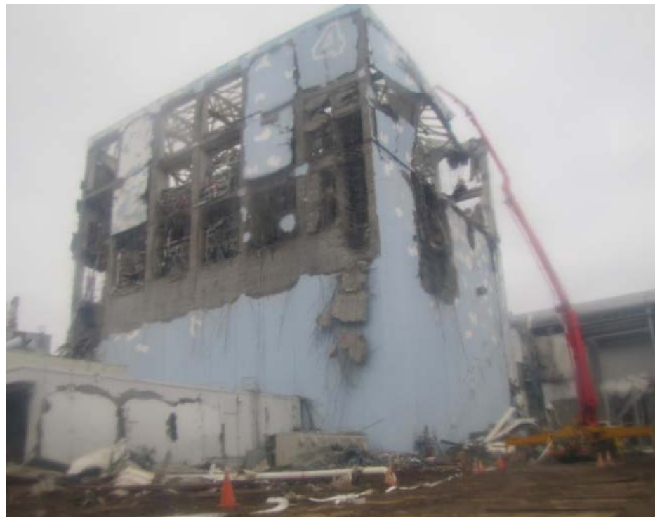
Photo: Water spray into the SFP in Unit 4 using concrete pump truck
